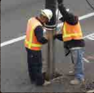
Key hole repairs
